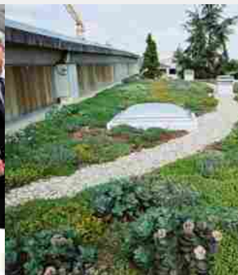
ENEA: a green rooftop to help regulate microclimate
